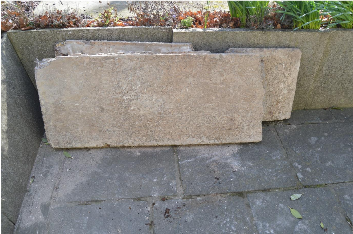
Figure 15: Concrete slabs that collapsed through the lead coffin lid. Here removed and propped up outside. Possibly part of a prefabricated concrete coal bunker.
