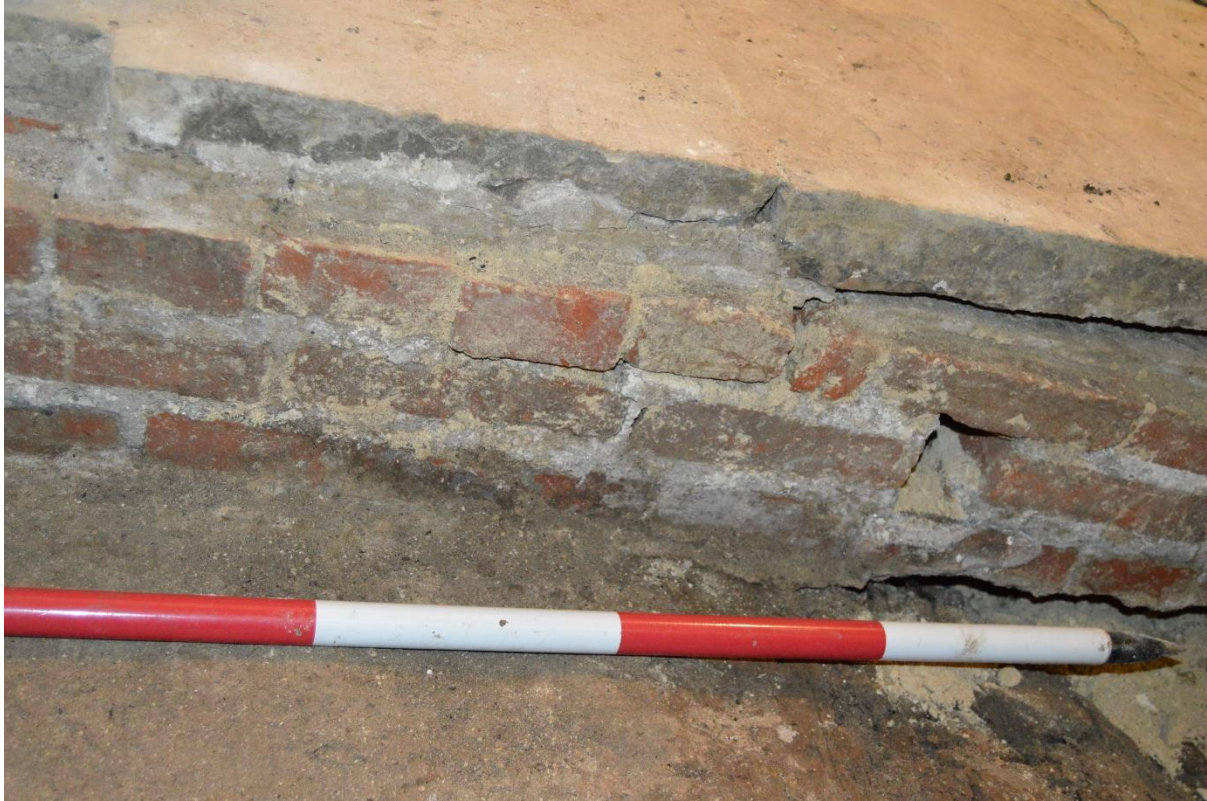
Figure 15: Northern sleeper wall built to accommodate the suspended limestone flag floor above.
