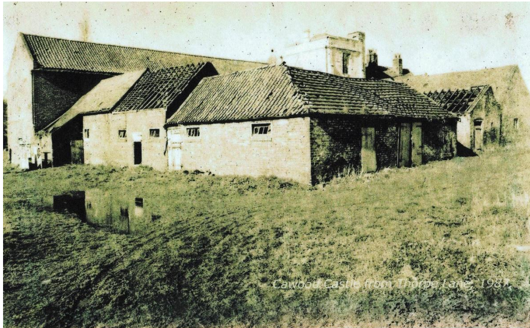
Figure 3: Image of Castle Farm buildings prior to demolition.
