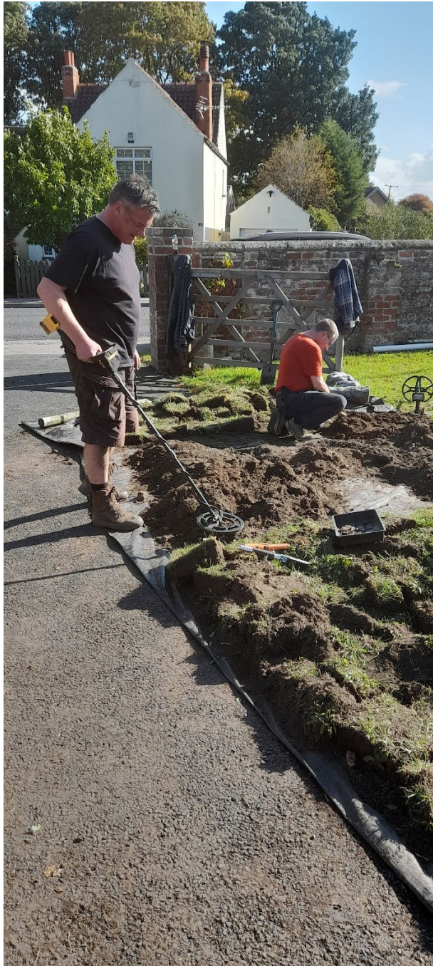
Detecting the spoil heap.
