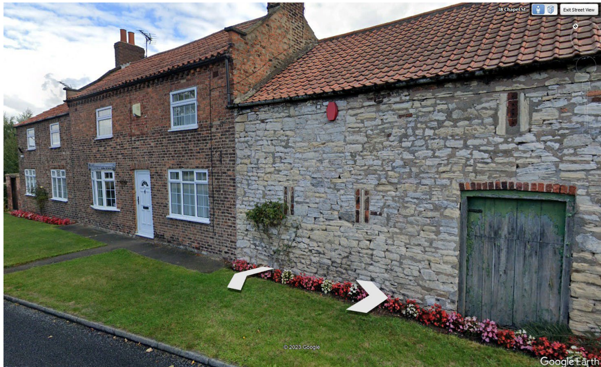
Figure 13: Hill Top Farm showing the stone foundations to the farmhouse and full stone construction to the barn. (Image Google earth Pro.)
