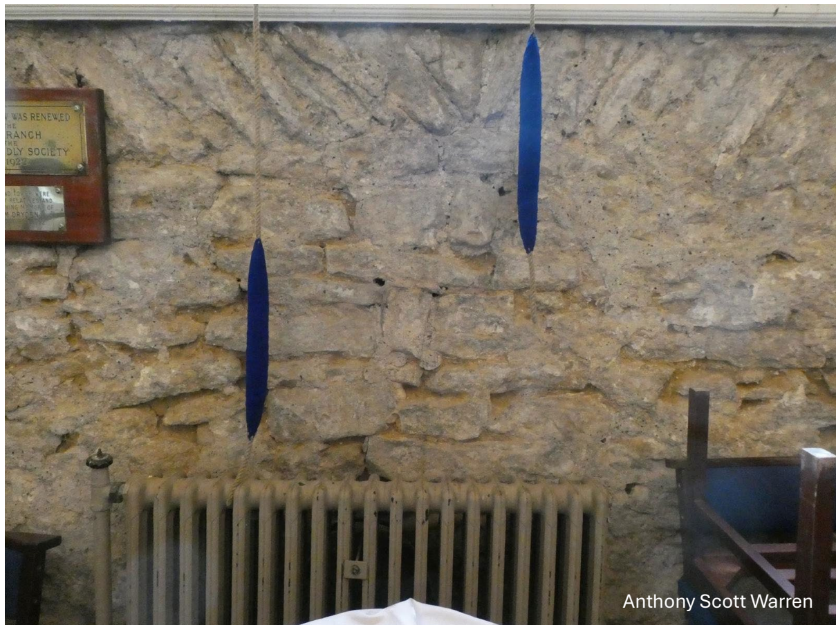
Figure 40: Rough stonework and herringbone at west end of St Mary's Church in Hook.
