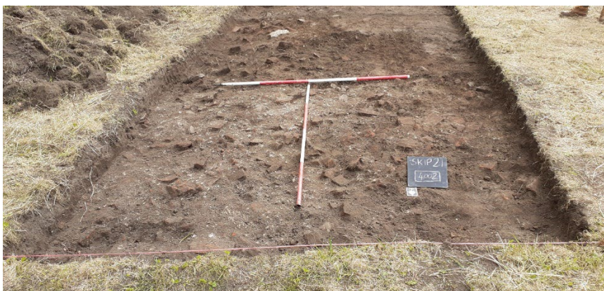
Figure 33: Demolition material covering structural remains in trench 4.
